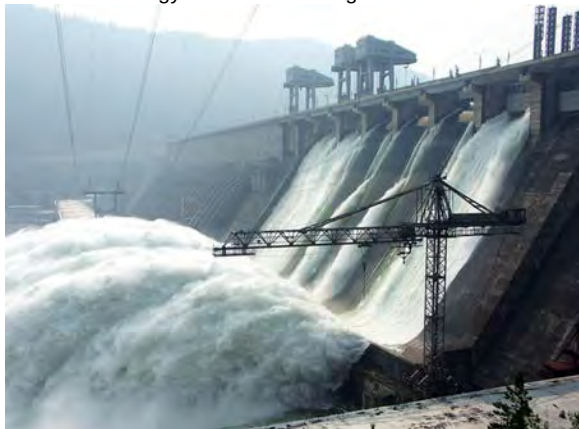
Figure 7.38 Hydroelectric facility (credit: Denis Belevich, Wikimedia Commons)
