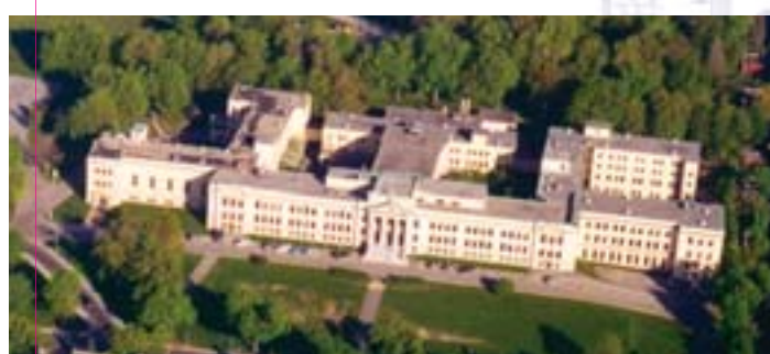
Aerial view of the new campus at 4873 Westmount Avenue.
